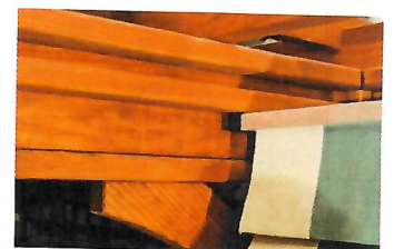
Side rails insure that the canopy stays level and true.
